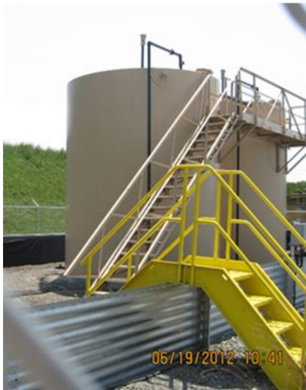
Figure B-12. Produced Water Storage Tanks
